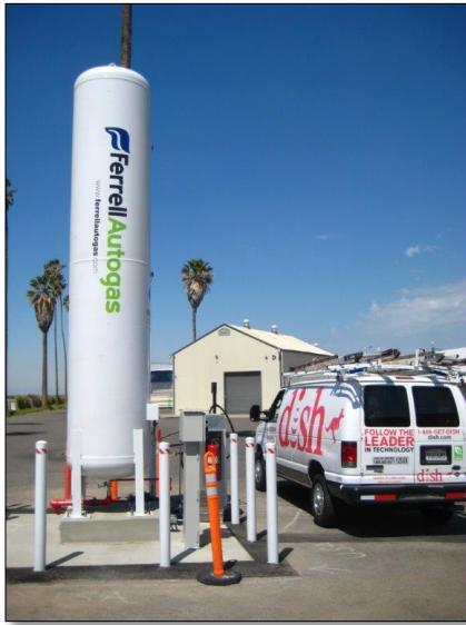
One (1) 1,000 Gal Vertical Tank
